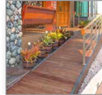
Example of porch and ramp.
